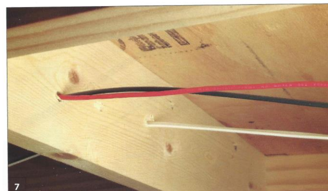
This shows the track bus wires twisted in the foreground and separated from the cab bus cable toward the rear. To avoid electrical interference, don't route the track and cab bus wires through the same hole.
